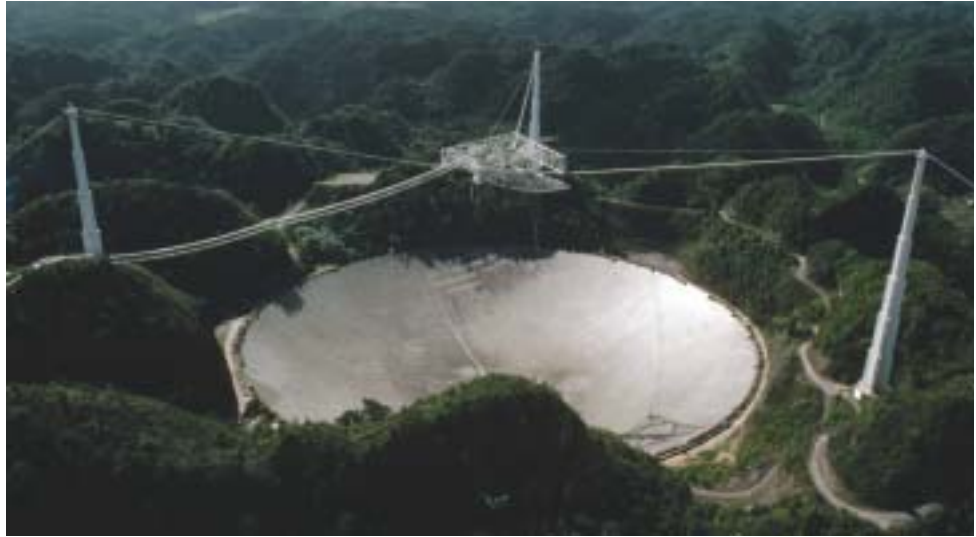
Figure 3.11 Because the wavelengths of radio waves are so large, the antenna of a radio telescope must be large. This radio telescope in Arecibo, Puerto Rico, has a diameter of more than 300 m. That's almost the length of three football fields laid end to end.
