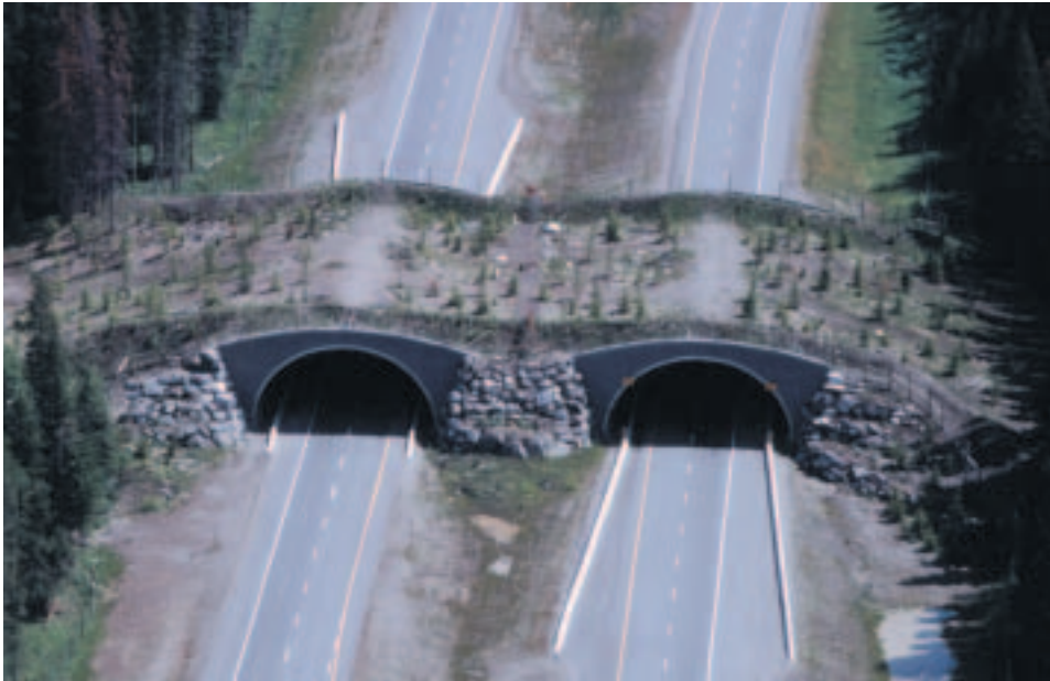
Figure 4.8 An aerial photograph of Redearth Overpass in Banff National Park
