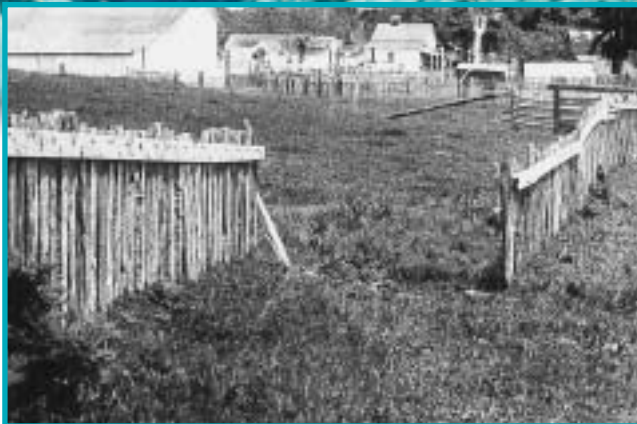
Figure 3.25 This fence was one straight piece when it was built. Why do you think it now has this gap?
