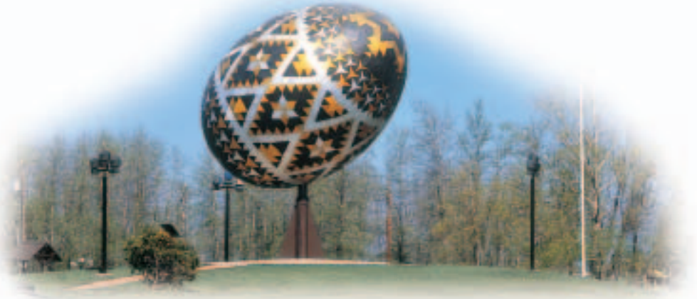
Figure 1.11 Honouring its Ukrainian heritage, the town of Vegreville built this monument to the pysanka (Ukrainian Easter egg). The aluminum egg, weighing 2270 kg and measuring 7 m by 6 m, stands on a steel and concrete base. Why might a concrete block with a plaque have been a less aesthetically pleasing structure?
