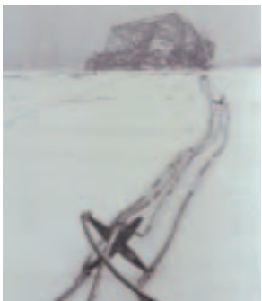
A downed hydro tower and power line, damaged by the 1998 ice storm in Quebec and Ontario.
