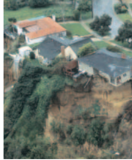
Figure 4.3 In Malibu, California, heavy winter rains during 1983 caused landslides on steep, unstable slopes. As a result, several homes suffered serious structural damage.
