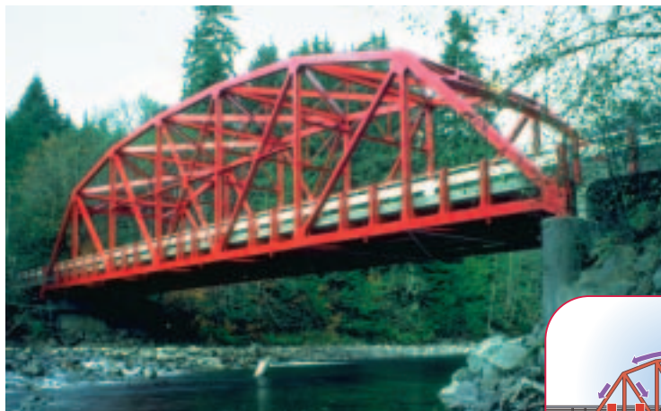
Figure 2.16 A truss bridge
