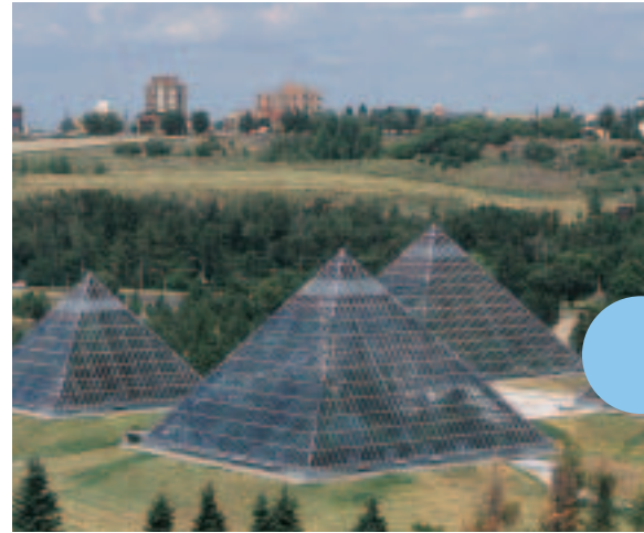
Figure 1.7 The Muttart Conservatory in Edmonton is noted for its five glass pyramids. Housed within these pyramids are indoor gardens that include tropical and desert plants.
